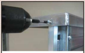
19. Install a DRILL POINT SCREW into each side of the shelf. The screw should go through shelf lip into the center of each SIDE MOLDING.
