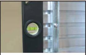
15. Stack up five more SLATWALL PANELS using same orientation as the first (Fig. 13). Tap sides with plastic hammer to align sides vertically. Tighten LONG PHILLIPS SCREWS on UPRIGHTS.
