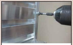
17. Attach LONG SIDE MOLDINGS (E) to the edges of SLATWALL PANELS. Install a DRILL POINT PHILLIPS SCREW (f) on each MOLDING on the back side, in the location shown.
