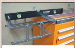
6. Check top of UPPER SIDE FRAME for level. Bend UPPER SIDE FRAME up or down if necessary to make level.
