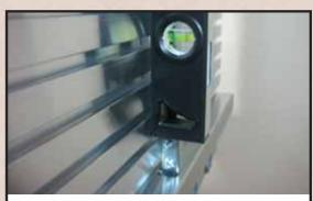
16. Check slatwall face for vertical and tighten HEX BOLTS and NUTS on UPRIGHTS.
