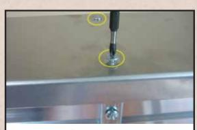
18. Place SHELF (F) on top of UPRIGHTS. Center SHELF side to side above SLATWALL. Slide SHELF all the way forward. Install two DRILL POINT SCREWS through top of SHELF into each UPRIGHT as shown.
